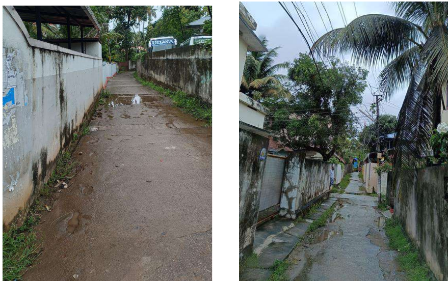
Fig 1.5: Location 8: Manichithodu - Completely covered with slabs in Peoples Nagar
