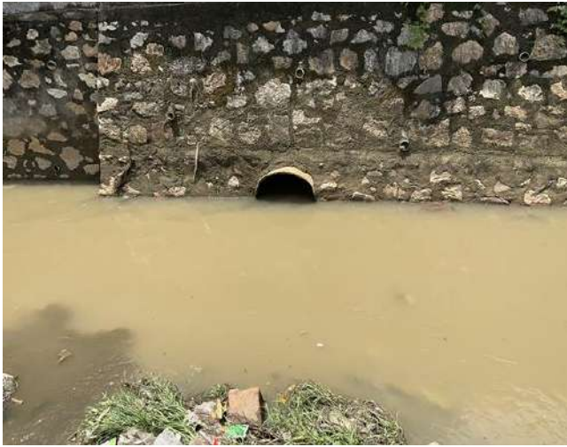
Plate 14: Overflow of sewage from Pattoor sewage pumping station in to the canal, drain/nallah
