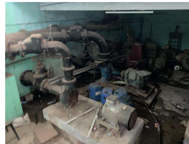
Plate 13: Pattoor sewage pumping station, pump not in working condition or scrab
