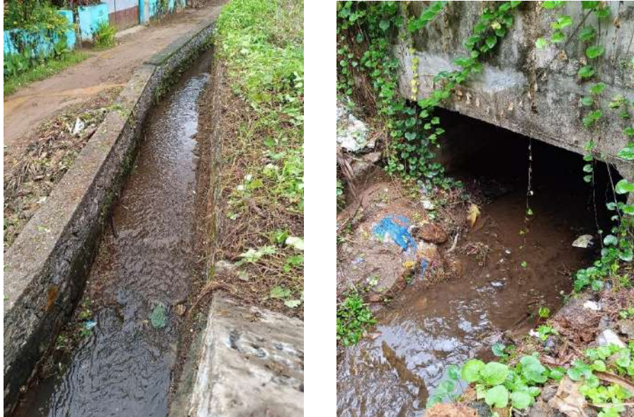
Fig 1.4: Location 4 & 5: Railway Culvert near Pattathanam and NTV Nagar
