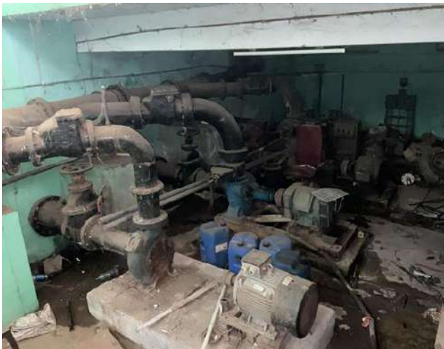
Plate 13: Pattoor sewage pumping station, pump not in working condition or scrab
